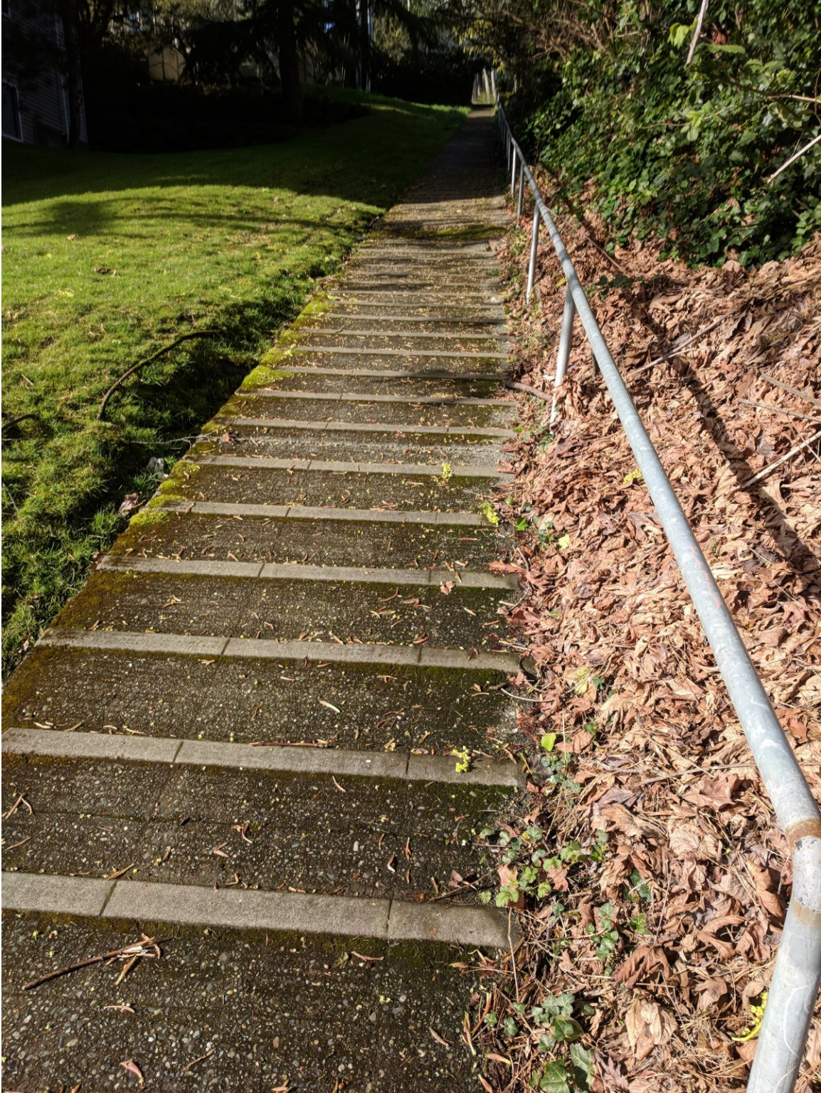
Figure 3: Existing Conditions Looking Southwest
